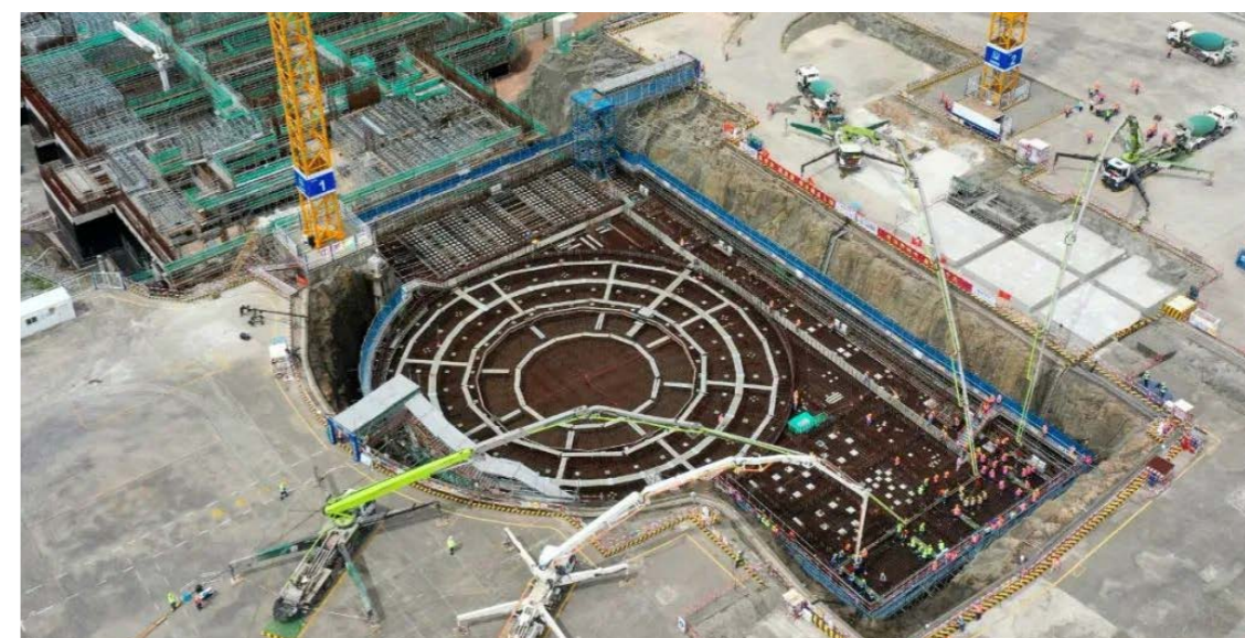
Sanmen Nuclear Power Plant Phase II Project
