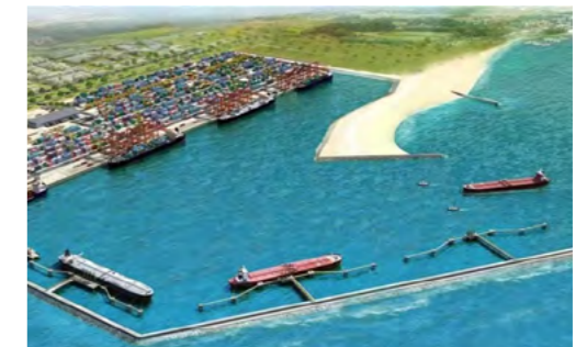
Panorama of the Lekki Port Project in Nigeria
